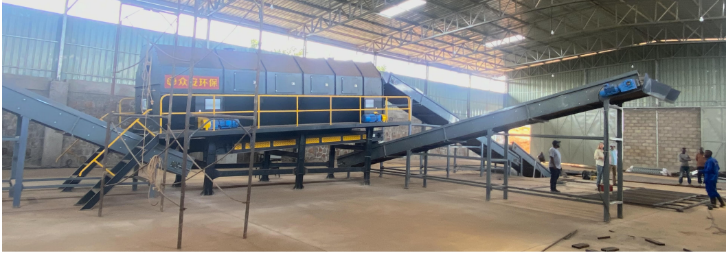
Figure 14: Construction in progress of the new sorting machine.
