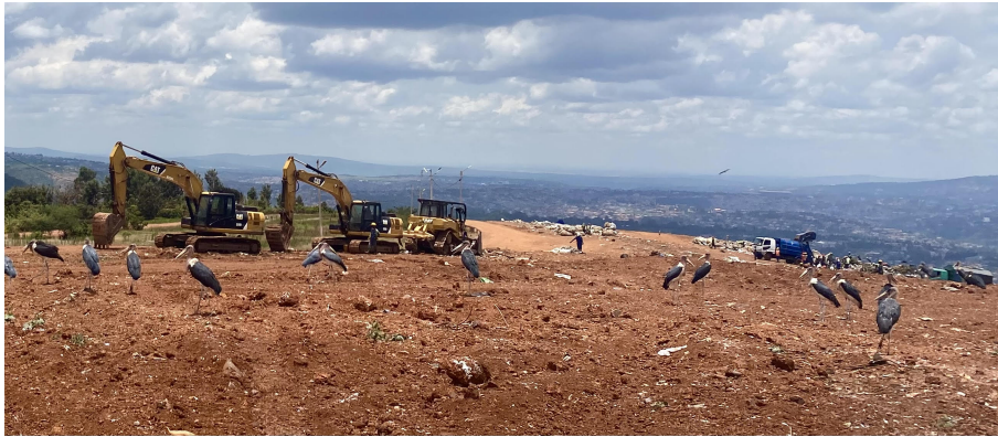
Figure 9: Machines spreading and compacting waste onsite. Marabou storks are common.
