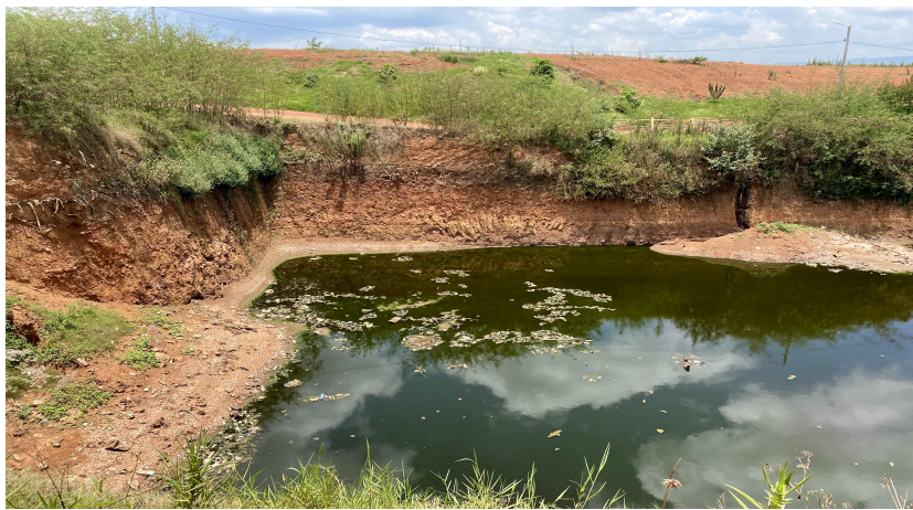
Figure 11: One of the three ponds designated for the storage of leachate water.
