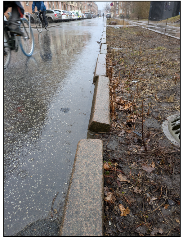
Figure 12: Water flowing into green buffer along Tåsinge Plads (photo taken by author)
