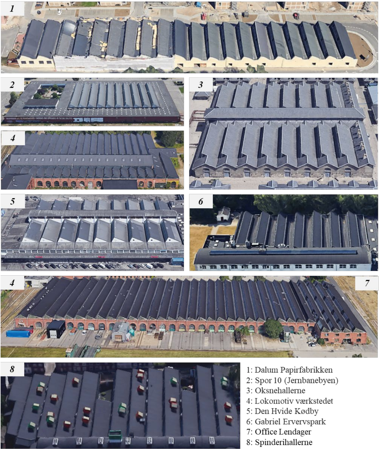
Figure 36: Single Floor, bi-axial building examples. Images taken from Google Earth (2025)
