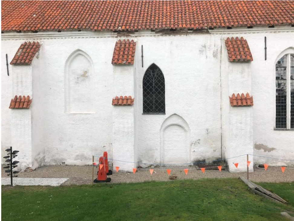
Figure 8. Bricked-up southern portal on S:ta Gertrud
