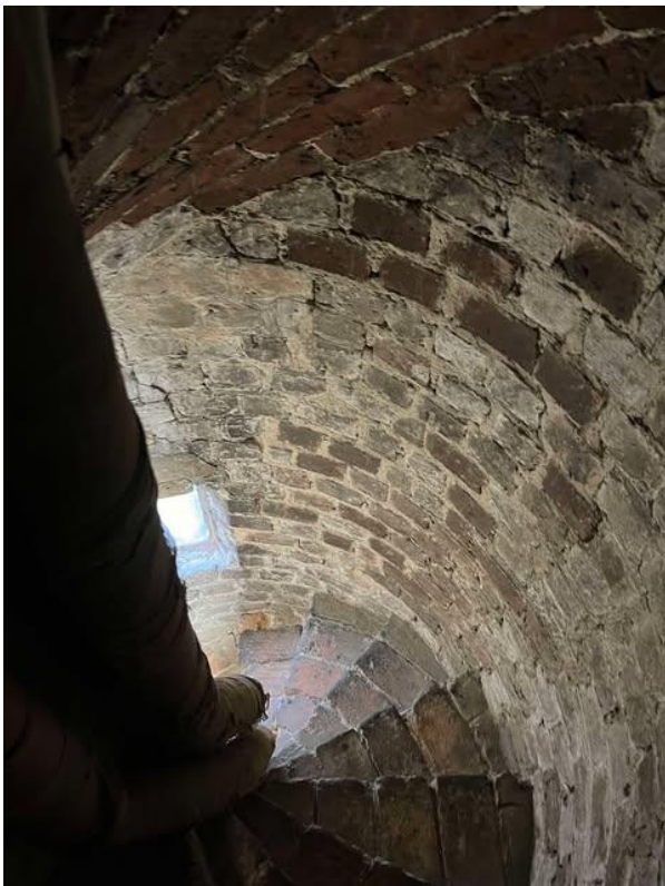
Figure 20. The oldest staircase in Malmö.
