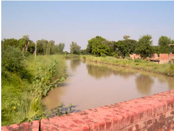
Figure 2: The Haidergarh canal Source : Photo by Author
