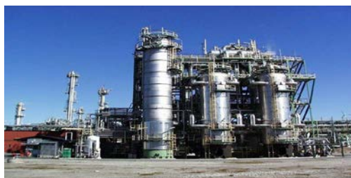
Picture 1. The Ethylene Oxide reactors at Akzo Nobel in Stenungsund
