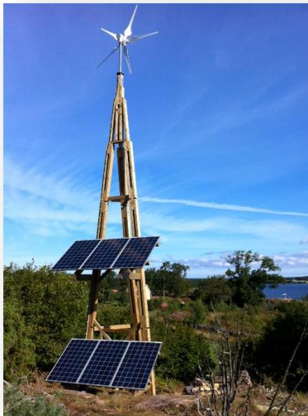
In the case of the purely renewable energy system, as well as the hybrid system, there was a need for over-dimensioning the systems in order to be able to meet the load more than 95 % of the time. By conducting a cradle-to-gate life cycle assessment study (including the diesel consumption) the environmental impact of these three energy supply systems could be calculated.
