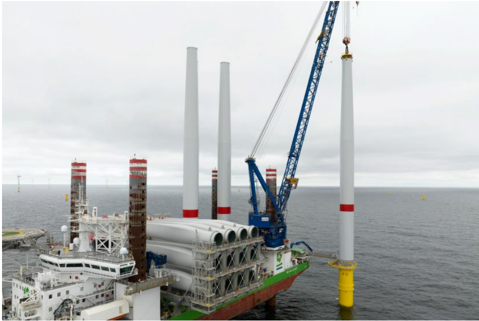
Figure 5: Installation of a tower (RWE Renewables n.d.).
