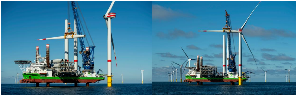
Figure 7: Installation of the blades (RWE Renewables n.d.).
