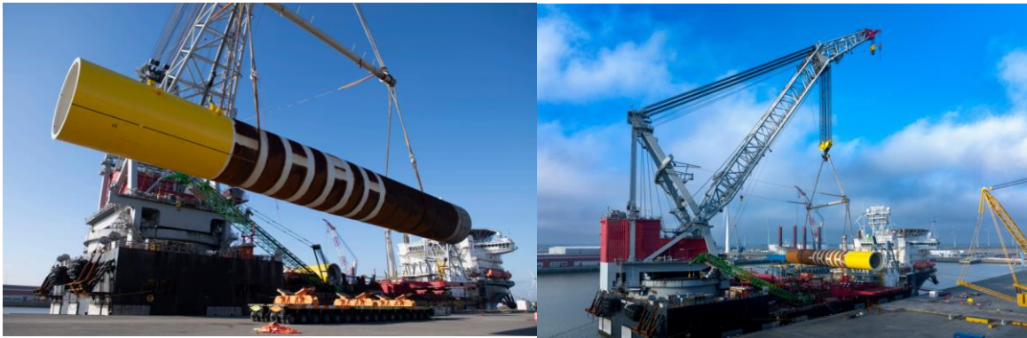
Figure 2: Monopile foundations are lifted onto a vessel (RWE Renewables n.d.).
