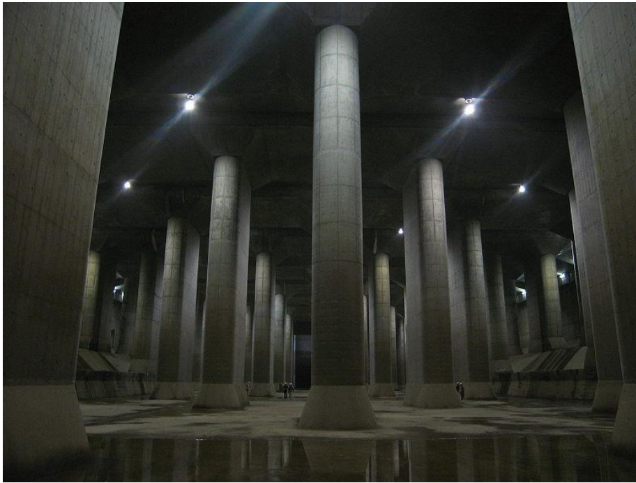
Figure 2-2: Metropolitan Area Outer Underground Discharge Channel. Kasukabe, Japan.
