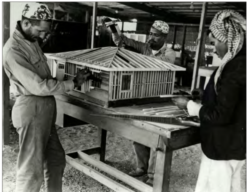
Figure 7. Saudi carpenters constructing a timber frame house model in an effort to fully understand its construction techniques and specifications. Photographer unknown, Courtesy of Saudi Aramco.
