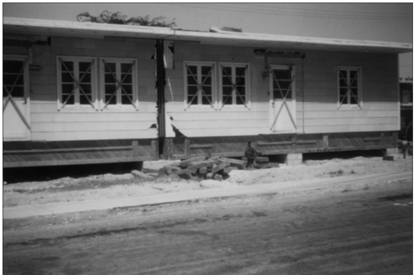
Figure 3. A Swedish duplex being prepared for relocating. Photographer unknown, Courtesy of King Abdulaziz Foundation for Research and Archives (Darah).
