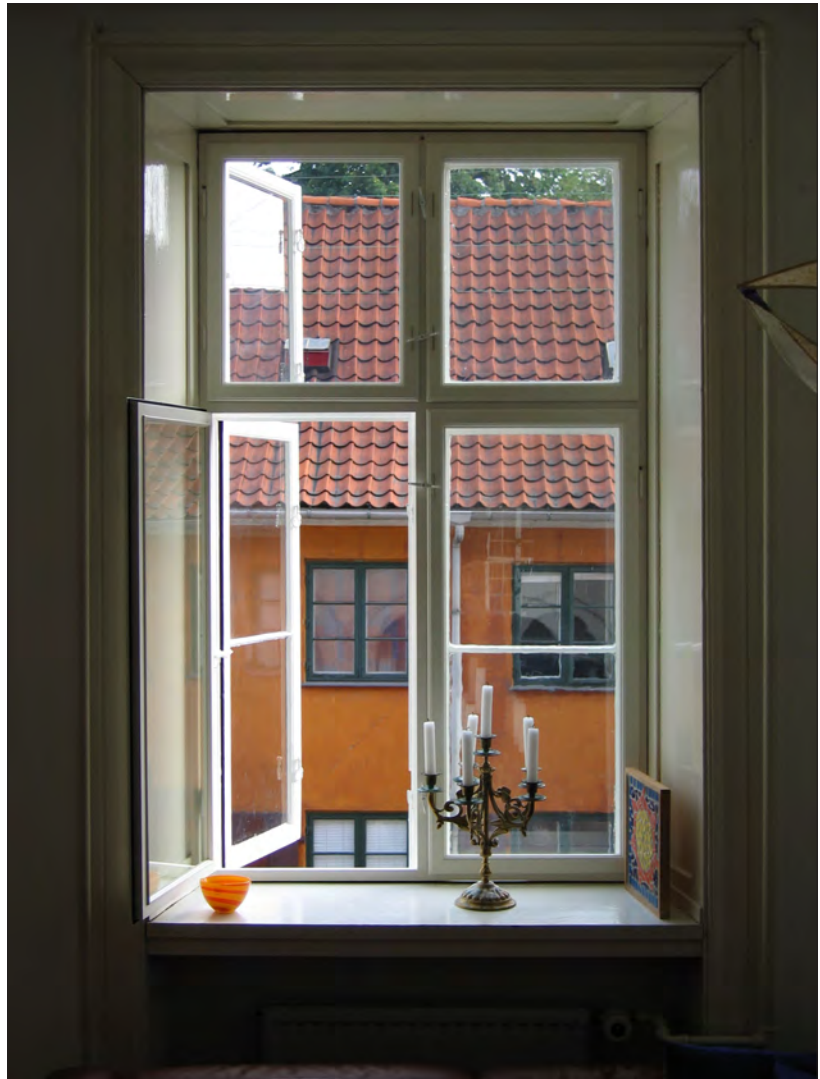
Figure 2. Typical Danish window with secondary glazing. Source: Thomas Kampmann.
