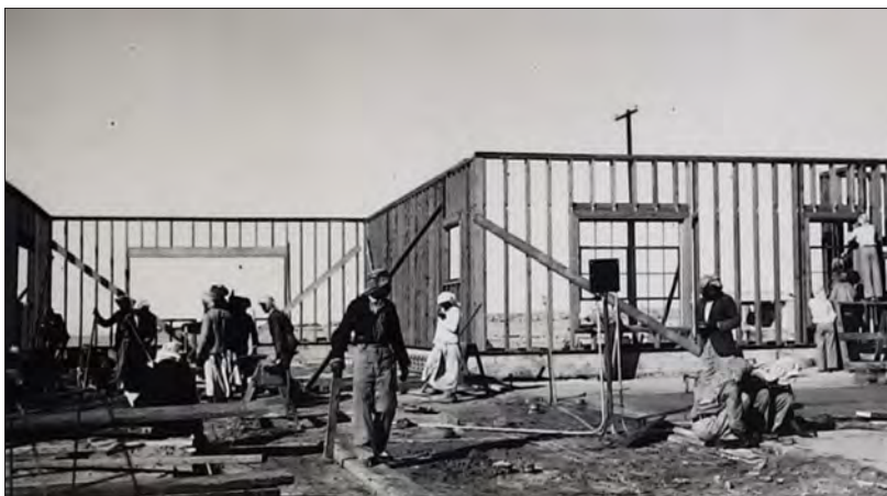
Figure 6. Saudi workers participating in a Californian timber frame construction in Dhahran camp in 1936. Photographer unknown, Courtesy of Special Research Collection, UC Santa Barbara Library, Saudi Arabia Oil Photograph collection, Bernath Mss 366.
