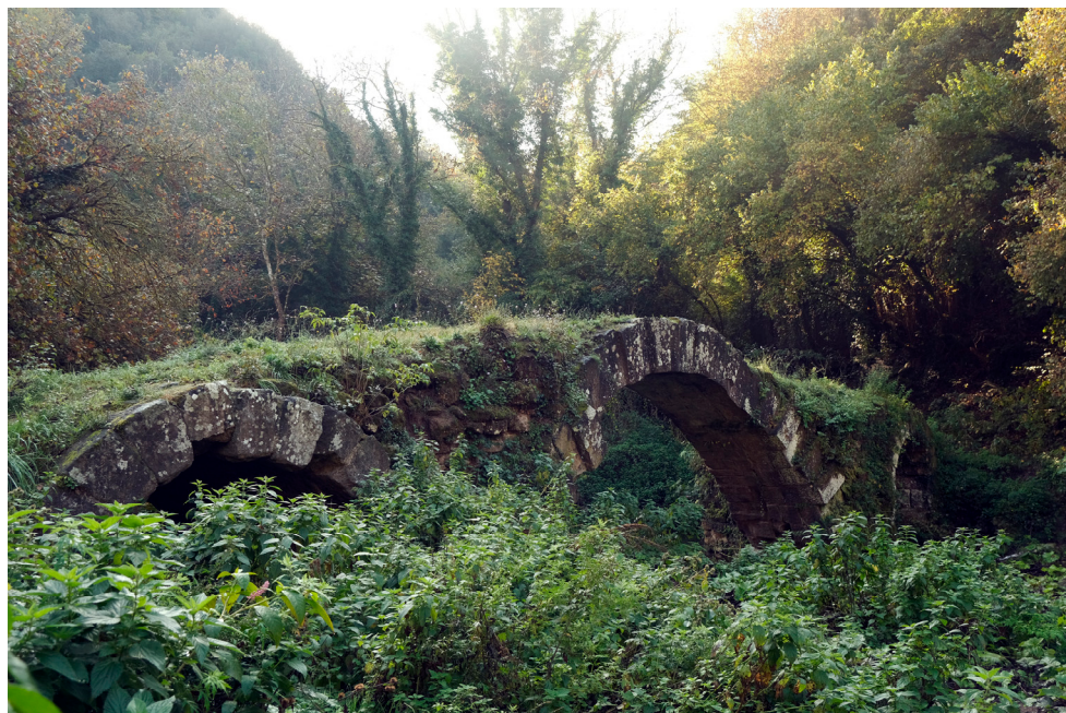
Fig. 19. Blera, Ponte del Diavolo (1st century BC). Photograph by R. Abedi.
