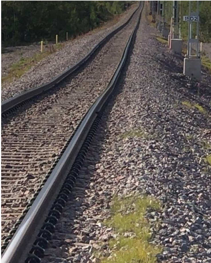
Figure 13. Track Settlement along Malmabanan Track, reprinted with permission (photograph: Tony Armstrand, Trafikverket)
