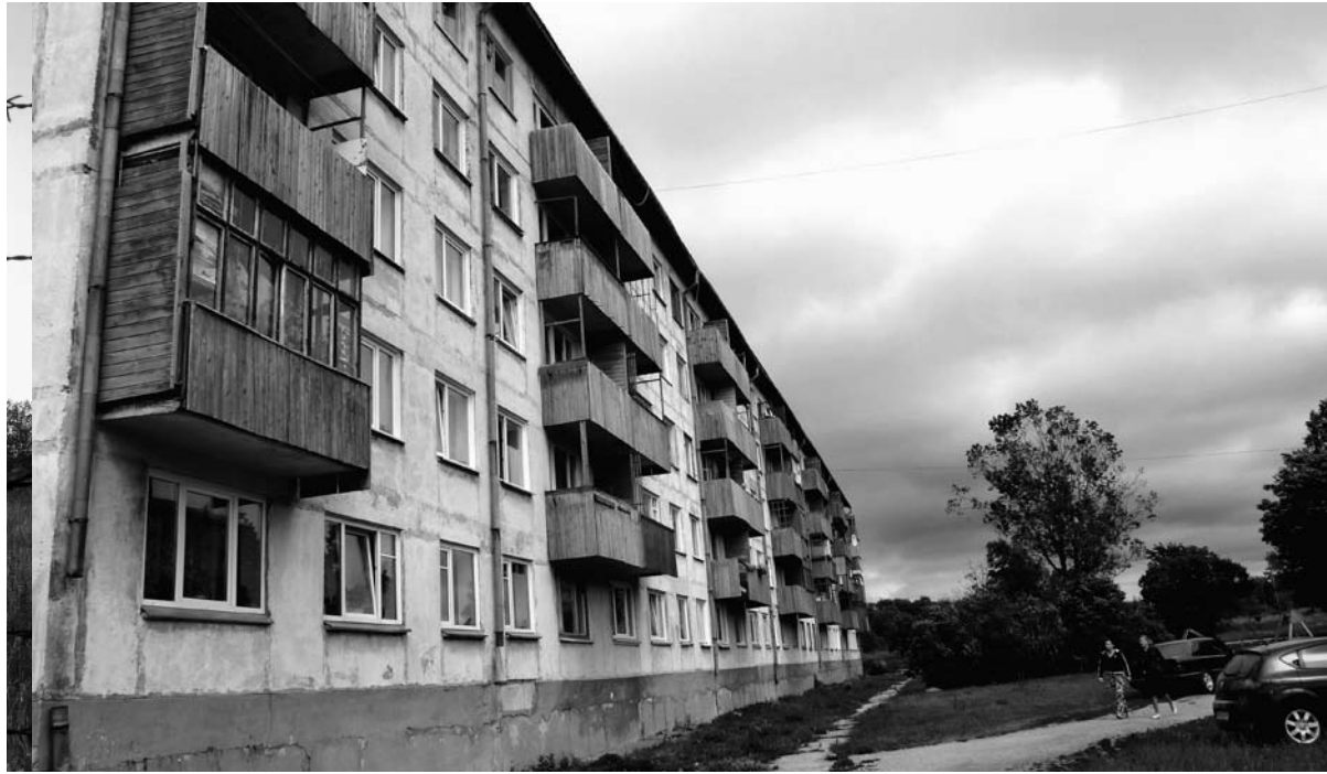
Paldiski – house with wooden balconies
