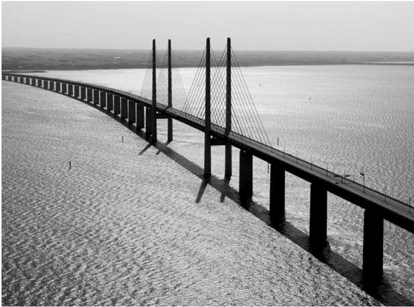
The Bridge across Öresund, from Malmö to Copenhagen, was inaugurated in 2000. Photo: Søren Madsen.
