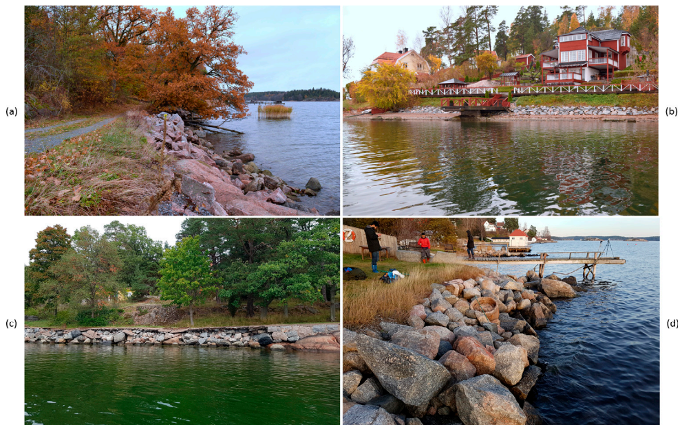
Figure 3-9. Examples of landowner initiative of erosion protection along the Furusund Fairway. (a) A rip-rap revetment is protecting a private road. (b) A seawall of rocks stabilizing the shoreline in front of a house. (c) A seawall that have been damaged by wave forces. (d) A rip-rap revetment protecting private property from eroding. (Photos taken in October 2016 (a-b), in August 2019 (c), and in December 2019 (d)).
