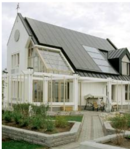
Figure 2. IEA5 Solar House
