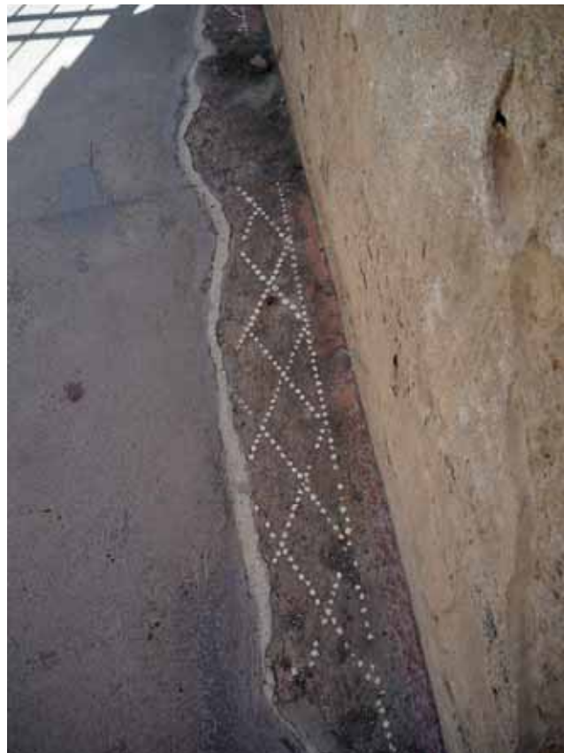
Fig. 71. Mortar-floor with a reticulate pattern in the fauces of Cd Octavius Quartio (II 2,2).
