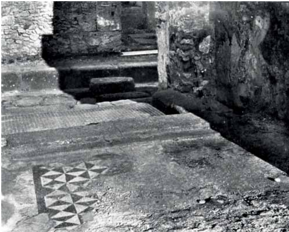
Fig. 77. Fauces -mosaic with hourglass-pattern in main section of the entrance in VI 13,13 (no. 8). View from atrium .
