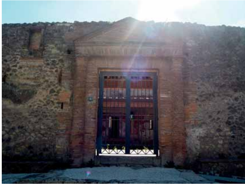
Fig. 39. Entrance to the semi-public bath-section of Praedia di Iulia Felix (II 4,1-12, no. 2).
