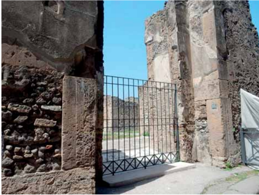
Fig. 19. Façade of Cd Aulus Umbricius Scaurus I (VII 16,12-13, no. 16), with a small recess in front of the door.
