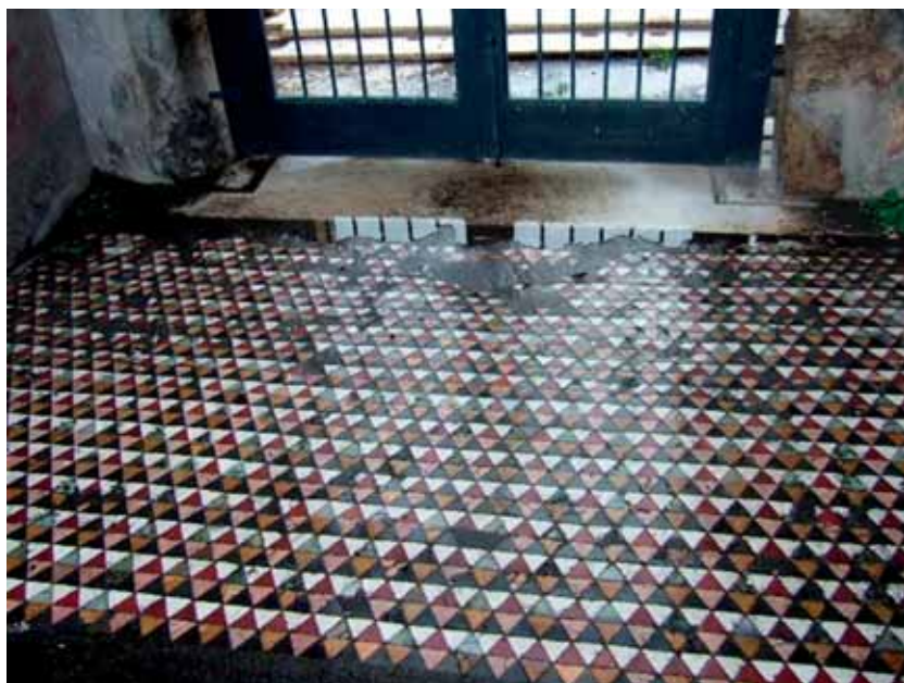
Fig. 32. Fauces -floor in Cd Fauno (VI 12,2, no. 7) in opus sectile -technique. View from atrium .
