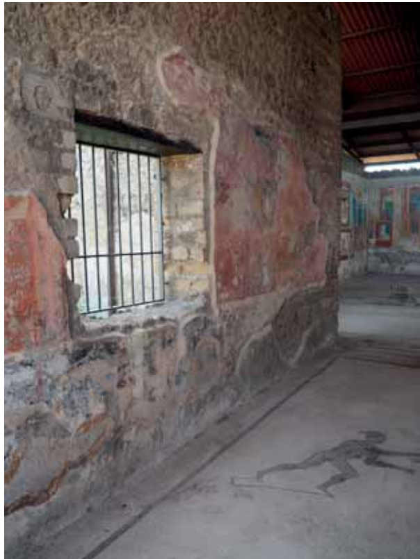
Fig. 146. Window between the adjacent taberna and the fauces of Palaestra (VIII 2,23, no. 22).
