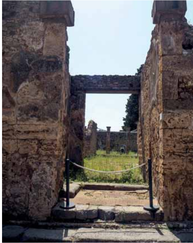
Fig. 7. The façade and portal of VI 13,13 (no. 8), providing a so-called Durchblick .
