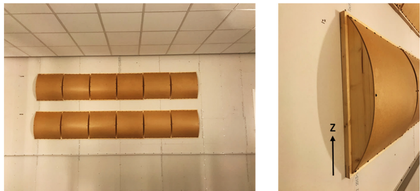
Figure 4. Vertically oriented diffusers; most of reflections will be sent in z-direction.
