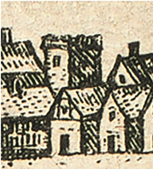
Fig. 13. Tower house in Lund, maybe the main building of the Bille Manor. Source/photo by Lund University Library, Alvin item no. 76516.
