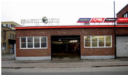
Figure 3.11. A building newly transformed into a garage in NGBG, 2009. Source: Norra Sorgenfi Nu Weblog.
