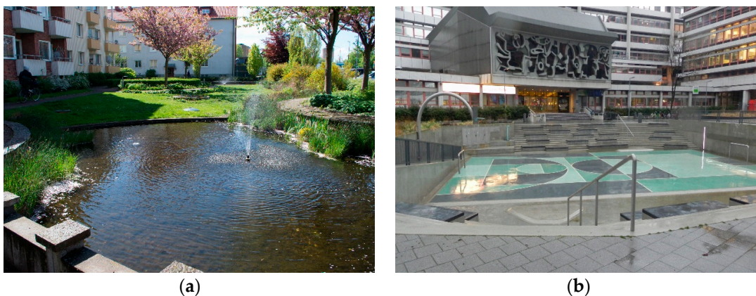
Figure 4. Floodable areas with multifunctional use. (a) A pond in Augustenborg Eco-City, Malmö. During heavy rainfall, the area can store water up to the stone edge near the trees to the right (photo by Johanna Sörensen); (b) The Water Plaza in Rotterdam. The multifunctional basins prevent surrounding streets from being flooded. The plaza is also used for performances, skating, studying, and group meetings (photo by Misagh Mottaghi).
