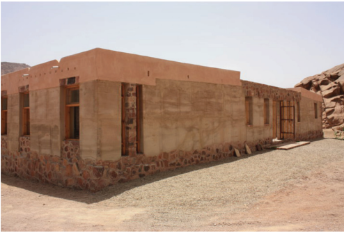
Figure 1. Using moulded earth and local stones showing the integration between local materials and the project site location. (Credits: Nashwa Ibrahim).
