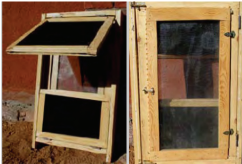
Figure 5. A window frame acting as a trombe wall using goat hair, where goat hair provides shading in summer and would act as a heat absorber in winter. (Credits: Ibrahim, 2011).
