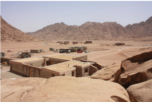
Figure 2. The layout of the project showing the choice of the site was based on climatic considerations. (Credits: Nashwa Ibrahim).
