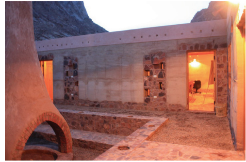
Figure 3. The courtyard as a main element in the design offering shaded and semi shaded areas for summer and winter use. (Credits: Nashwa Ibrahim).
