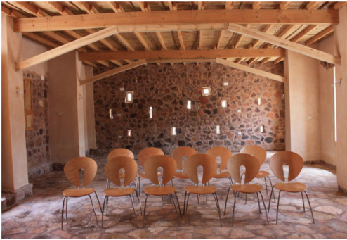
Figure 4. Different opening sizes inspired from ventilation and natural indirect light solutions in Saint Catherine vernacular buildings. (Credits: Nashwa Ibrahim).
