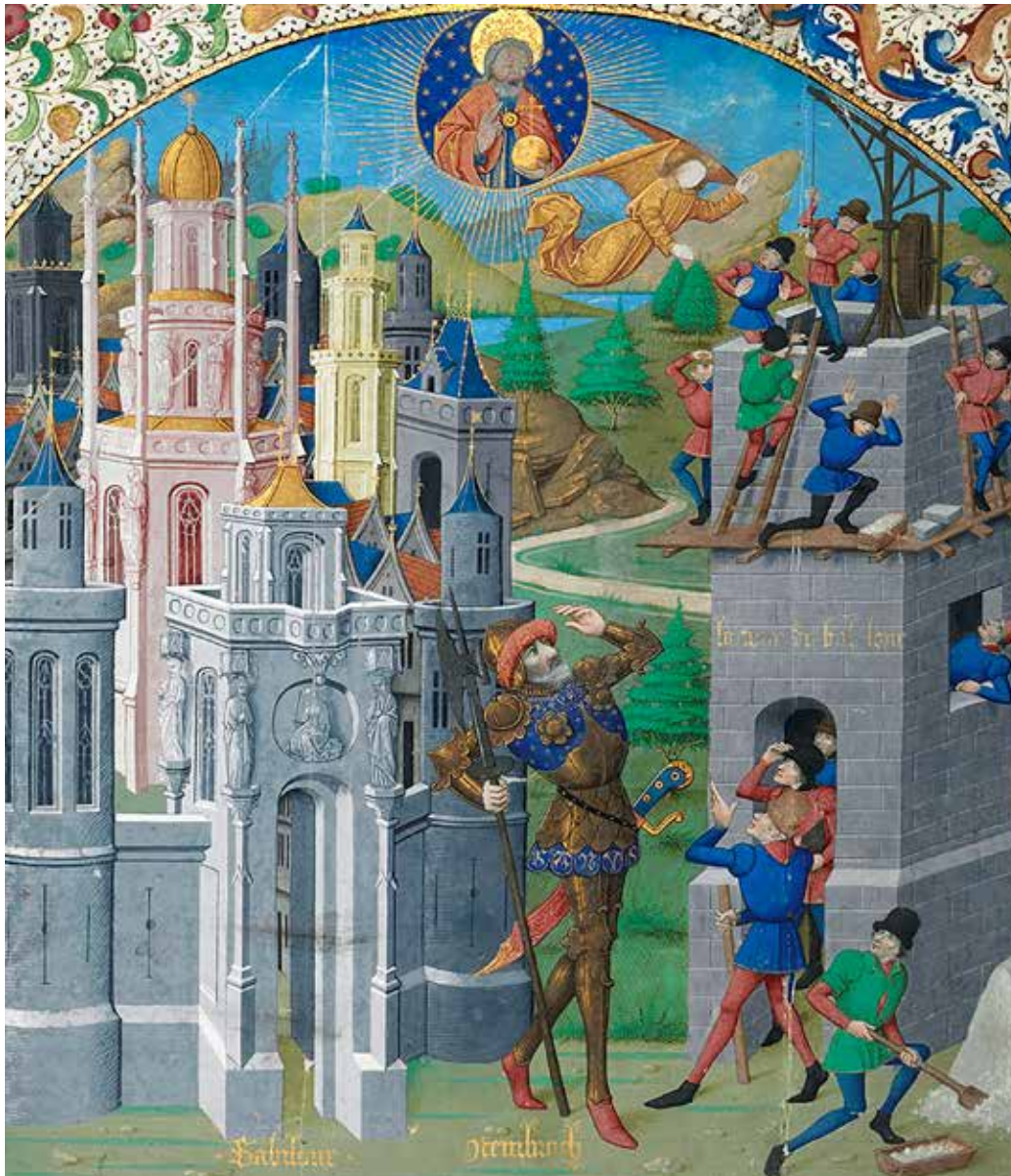
Illustration from the French book Chronique de la Bouquechardiére by Jean de Courcy from the end of the 1400s, showing the building of the Tower of Babel. The image shows the use of the same type of scaffolding as when Kärnan was built.
