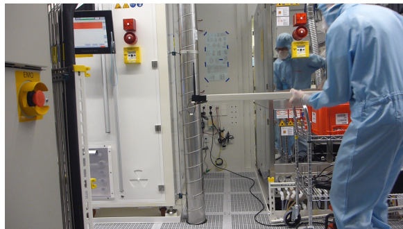
(c) View towards the left aisle.
