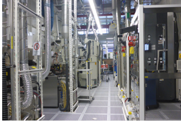
(a) View towards the co-located array.
