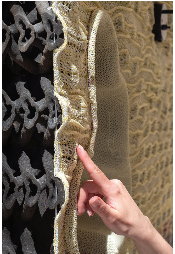
11 Fabric is fixed using integrated hooks and nylon threads
