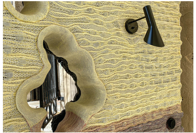
6 Light fixtures and cabling integrated into the 3D-printed structure
