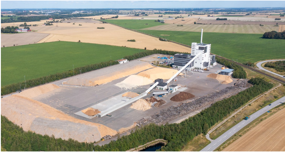
Figure 4. The Örtofta CHP plant. Photo: Peter Duvander, Krafringen Energi AB.
