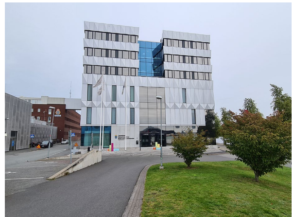
Fig. 14 Even a quite small district courthouse, such as the one in Jönköping (from 2000), has a certain monumentality to it. The old police building is on the left. Photo by author 2021
