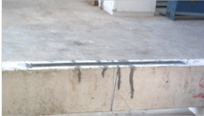
Fig. 8. Application of CFRP laminate for beams in group RF.
