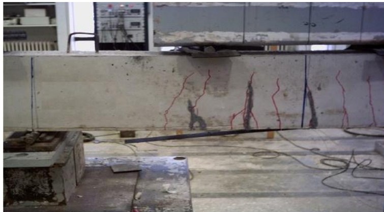
Fig. 15. Debonding failures in group RF.
