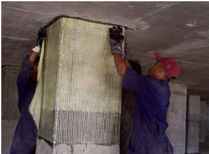
(b) Seismic retrofit of supporting columns for a cryogenic tank in Gujarat, India.
