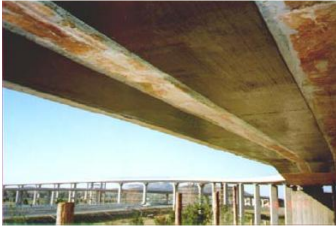
(a) Flexural strengthening of a highway RC bridge slab in China.
