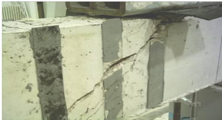
Fig. 18. Debonding and shear failures in group RS.
