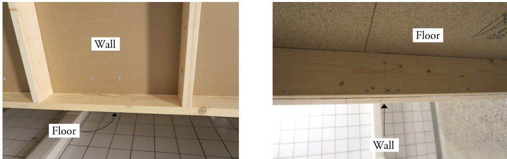
Figure 2.9: Photographs of a junction between the floor and a wall in the upper room. In the left photograph, the floor cannot be seen, but the arrow indicates its placement.
