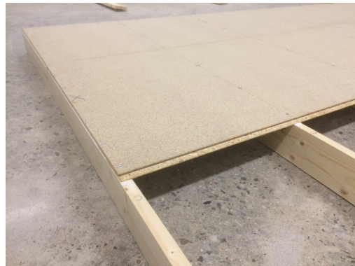
Figure 2.5: Photograph of the floor during mounting of the particleboards.
