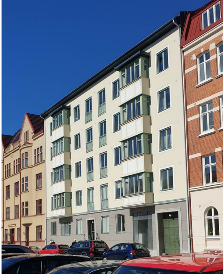
Fig. 17. Photo of Building 1 which is a 6-story residential building containing multiple apartments located in central Malmö, Sweden. Photo: Erik Kimblad.
