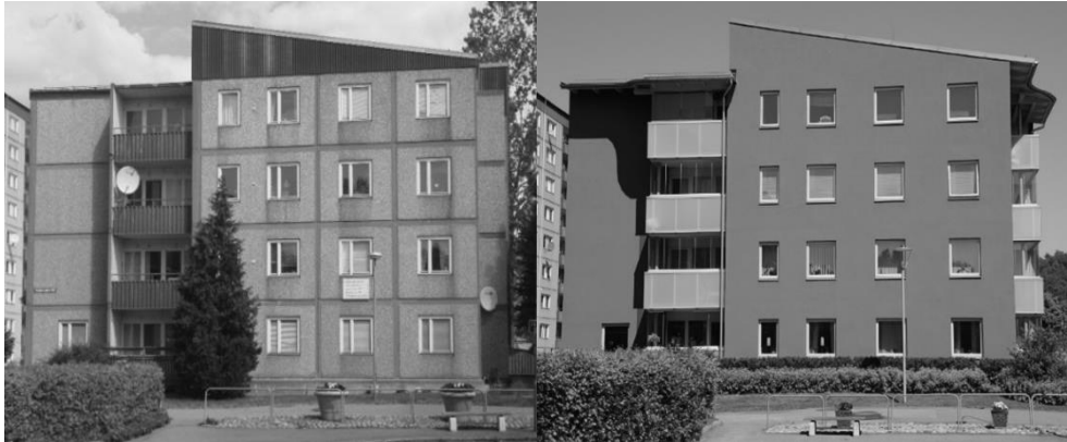
Figure 4.1 Photograph taken before (left) and after (right) the renovation. Photographs taken by Åke Blomsterberg.
