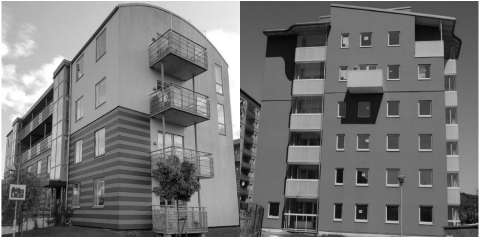
Figure 4.2 The two realised vertical extension projects. Photograph taken by Rikard Nilsson and Åke Blomsterberg.
