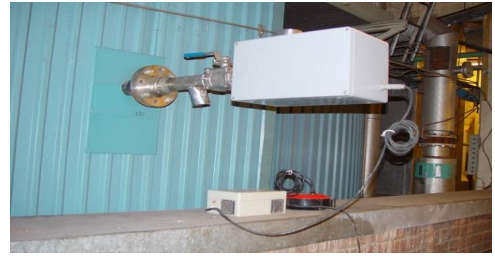
d. The transmitter mounted on the research CFB boiler.
