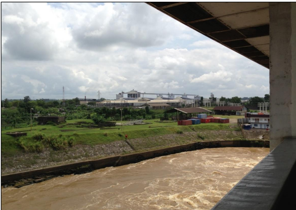
View of the aluminium smelter Alucam from the Edea hydroelectric plant, Cameroon.
