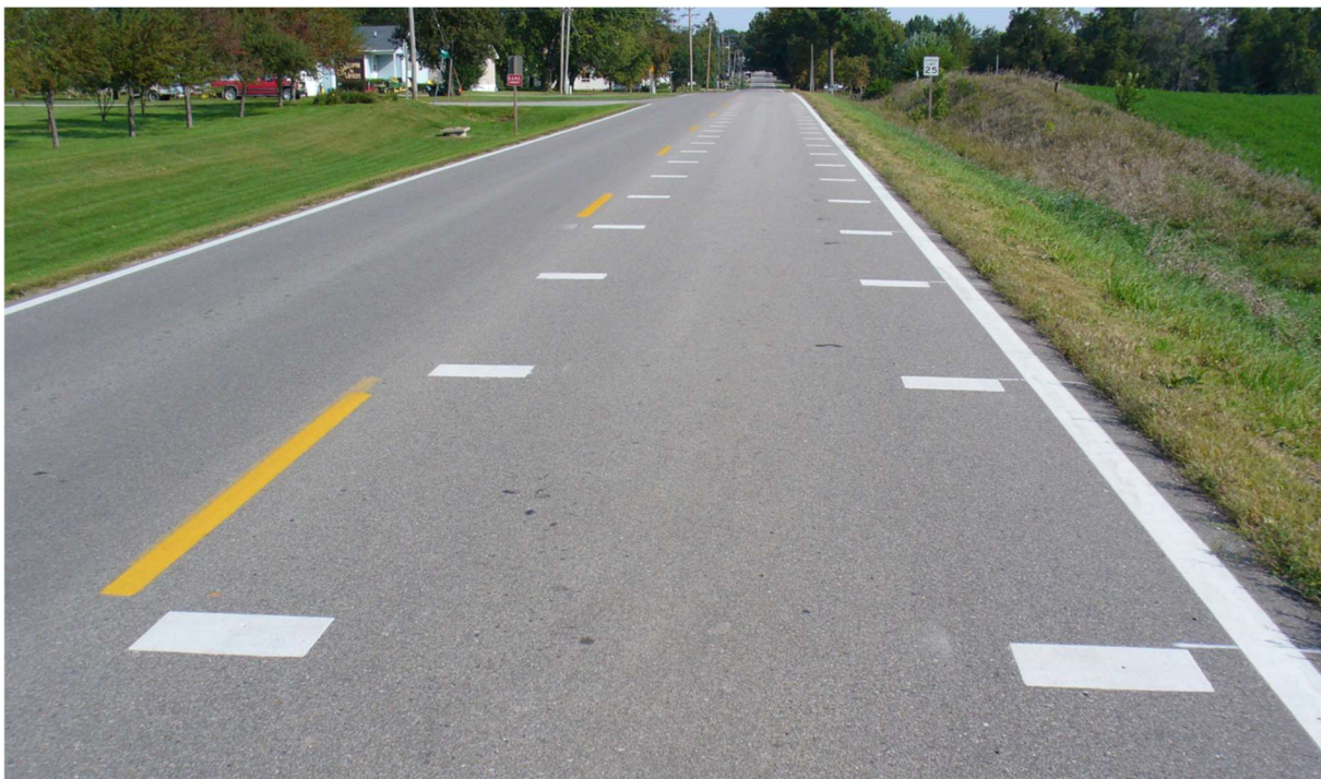
Figure 16. Transverse pavement marking bars (Fitzsimmons et al., 2009).
