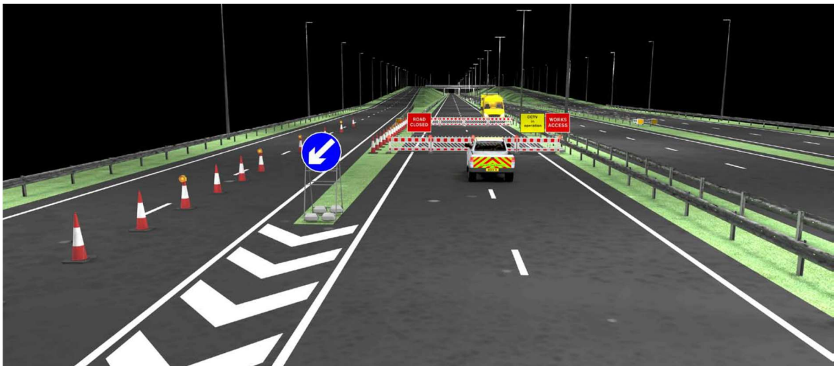
Figure 24. The ‘Airlock’ system at a complete carriageway closure (Highways England, 2016).
