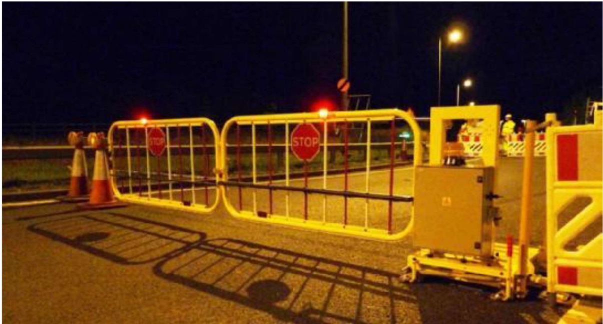
Figure 25. Automatic Gate to control access to the airlock (Highway Safety Hub, 2018).
