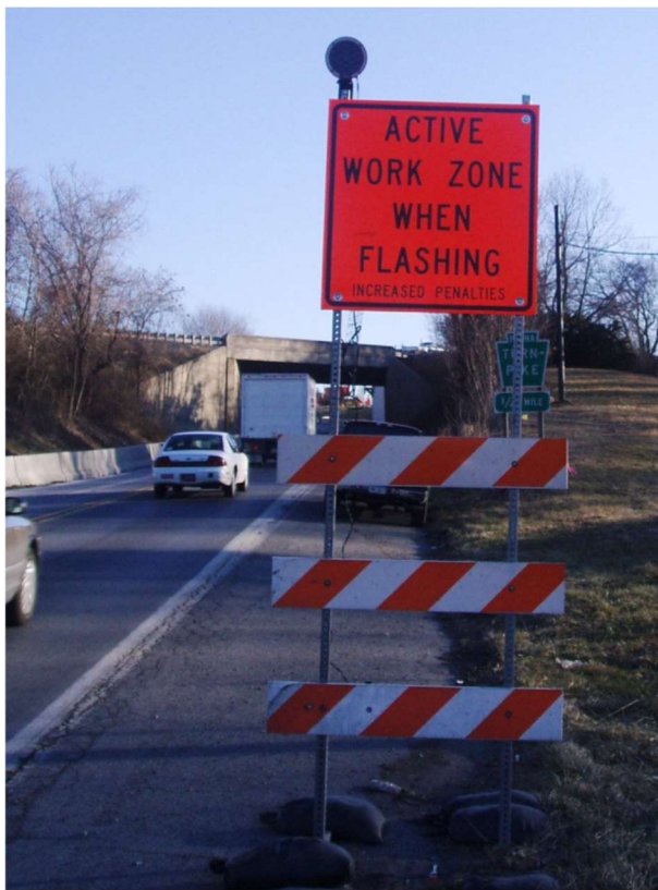
Figure 10. Work zone sign complemented with flashing light when road workers present at the site (Sesny, Lentz and Rensel, 2007).
