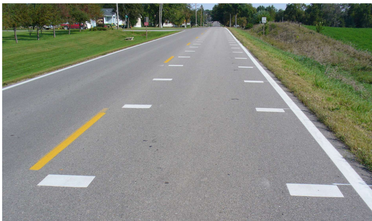
Figure 16. Transverse pavement marking bars (Fitzsimmons et al., 2009).
