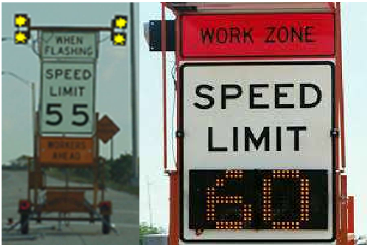
Figure 11. A static speed limit sign with flashing beacons when reduced speed limit is in effect and a variable speed limit sign at road work zone.
