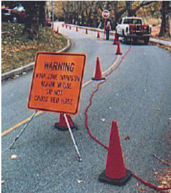
Figure 28. Pneumatic tube incursion alarm (Wang et al., 2013).
