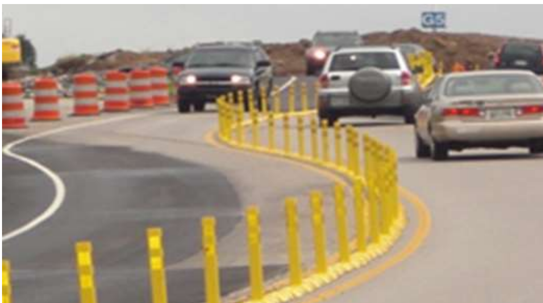
Figure 7. Curb system ( http://www.pexco.com/markets/industrial/traffic/lane-separator-curb-systems/fg-300-interstate-grade-curb-system/ )
