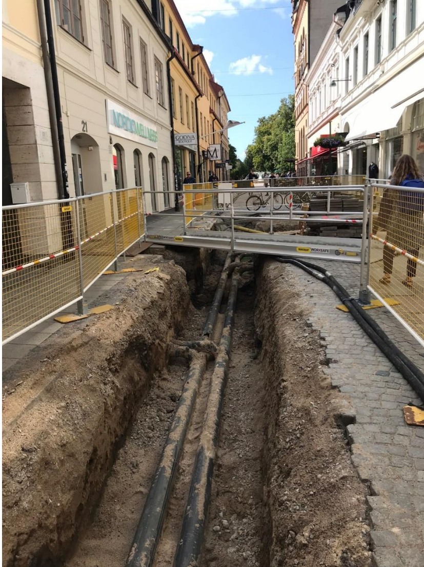
Source: District heating pipeline maintenance, Lund. Copyright: Aimee Ambrose.
