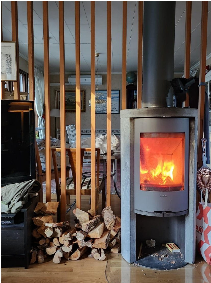
Source: Wood stove with Air Source Heat Pump in the background, Sweden. Copyright: Jenny von Platten.
