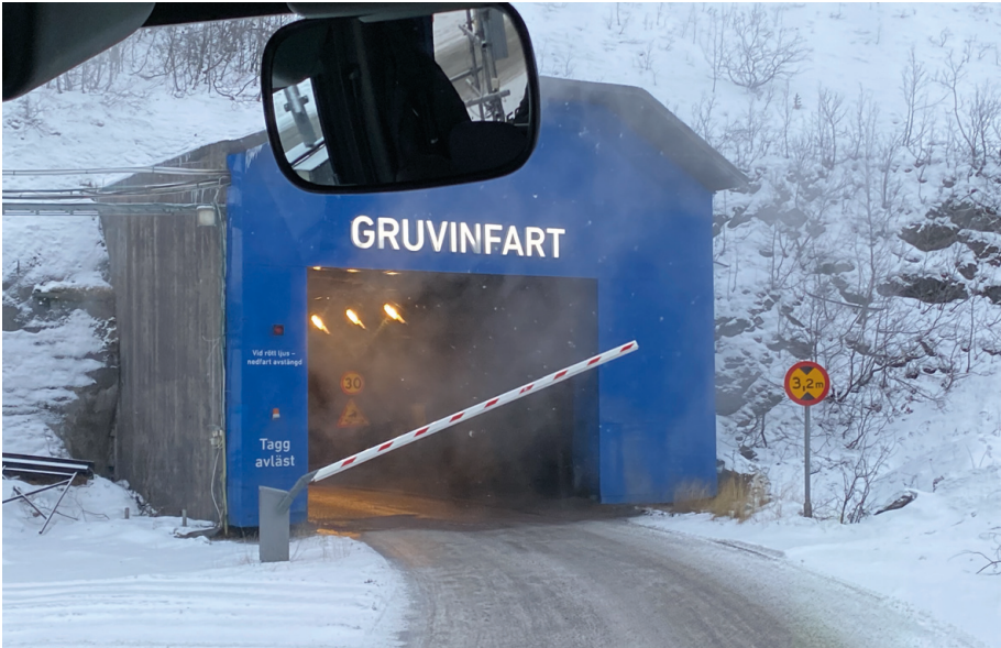
Figure 13. Approaching the Kiruna mine entrance by bus during a tourist tour. (O11)
