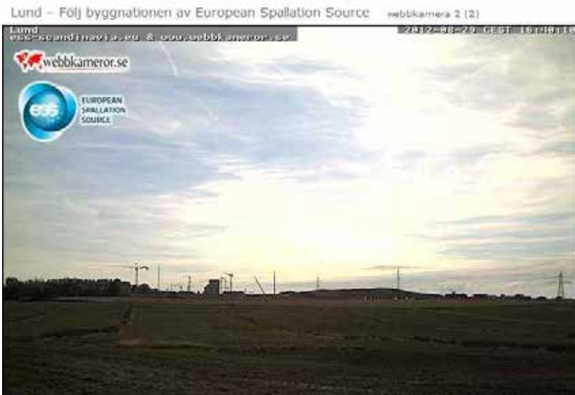
Figure 21. "Lund – Follow the construction of European Spallation Source". Photograph webbkameror.se
