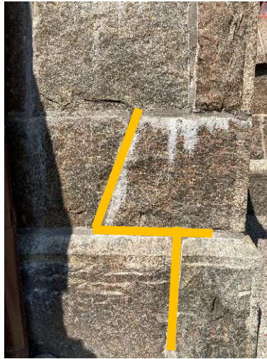
Placering fogbruk 8: hydraulisk Ortho-kalk.
