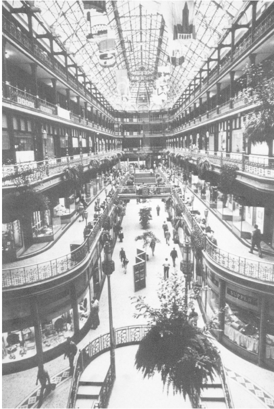
Figure 1.7 Arcade, Cleveland, Ohio, 1888-1890 (Saxon, 1983).
