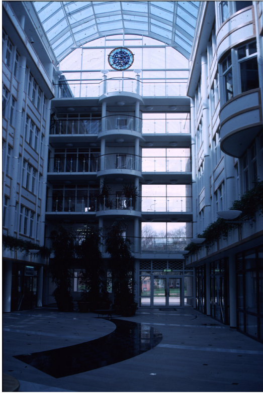
Figure 5.33 Interior of the office complex Scandinavian Center in Malmö (Wall & Blomsterberg, 1994).
