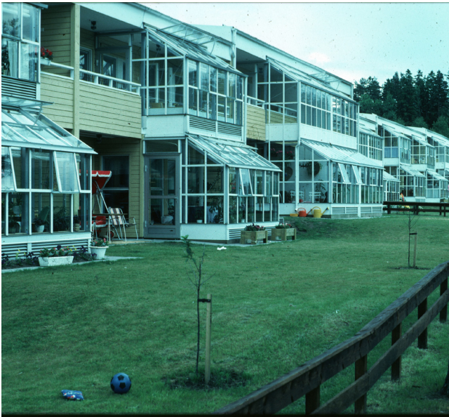
Figure 5.5 The south facade with its characteristic glazed verandas (Fredlund, 1995).
