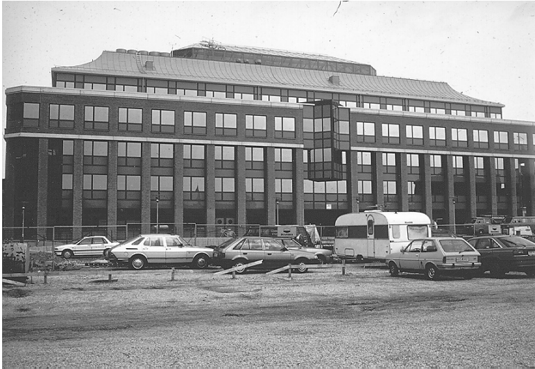
Figure 5.36 The office building Siriushuset in Malmö (Wall & Blomsterberg, 1994).
