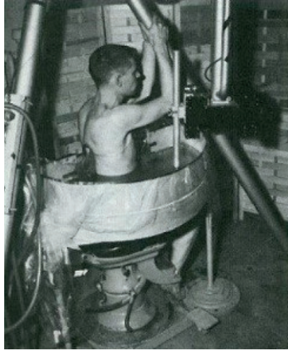
The Howry team's "pan scanner," developed c. 1957–1958. The patient sat on a modified dental chair strapped against the plastic window of a semicircular pan filled with saline solution, while the transducer rotated through the solution in a semicircular arc around the patient. A great many clinical scans were performed with this scanner, which was more appropriate for patient use than were the earlier total immersion scanners. Photo credit: The image originally published by Kodak Health Sciences and courtesy of the American Institute of Ultrasound in Medicine (AIUM) historical archive.
