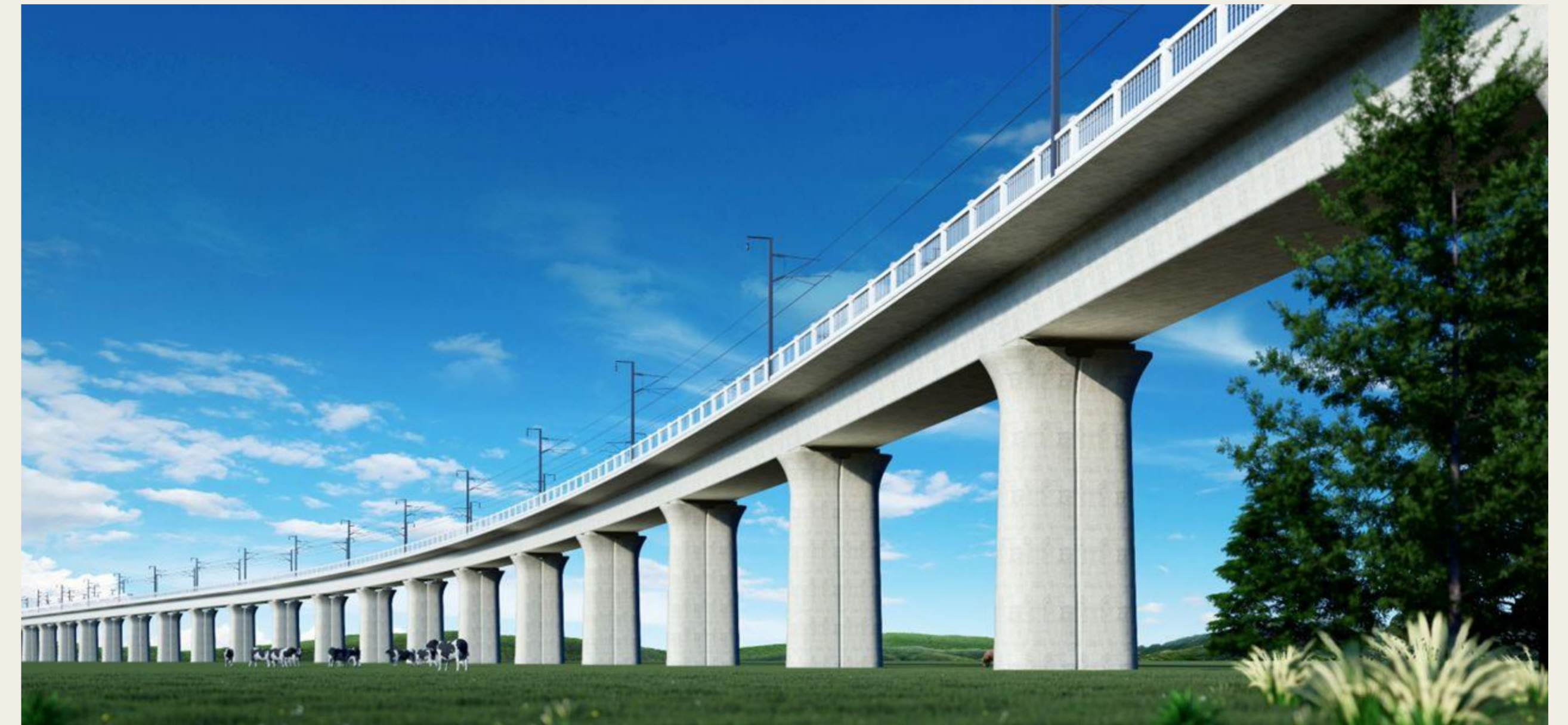
Fig. 1: Example of piers for the construction of high-speed rails.
