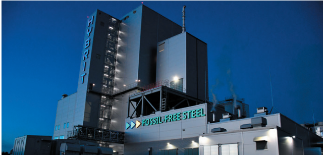
HYBRIT direct reduction pilot plant, Luleå
