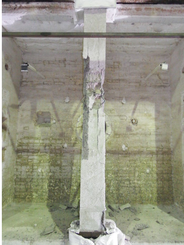
Fig 8. One RC column in the furnace after the test.
