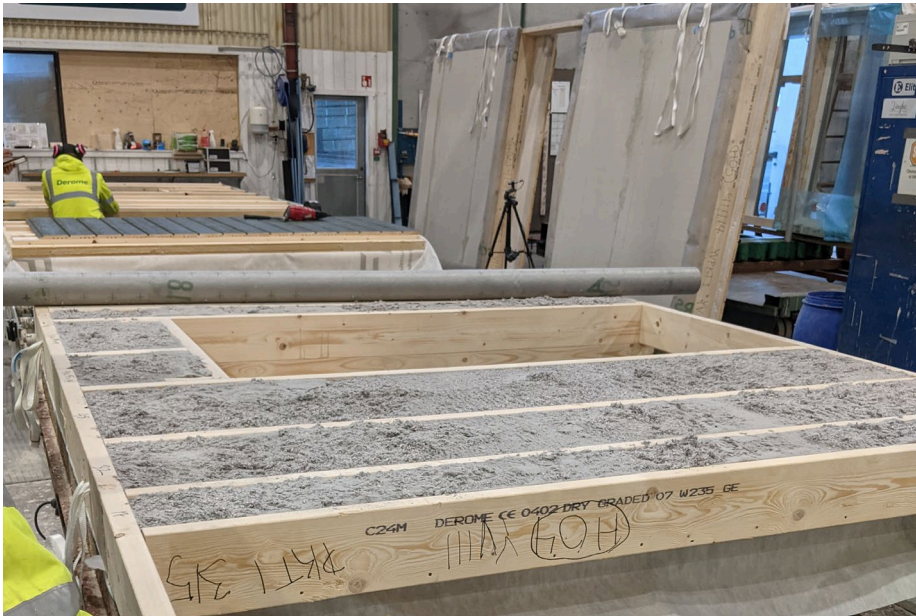
Figure 44: Wall element insulated with cellulose loose-fill for a test house by DEROME/A-hus.
