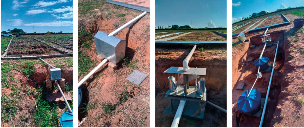
Figure 3.10: Photographs of tipping buckets installed on study area for real time runoff monitoring.
