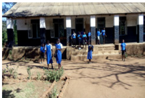
Pic 1. Domasi School steps before intervention.
