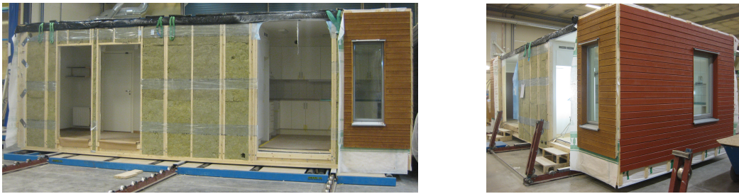
Figure 2.3: A TVE ready for transportation to construction site.
