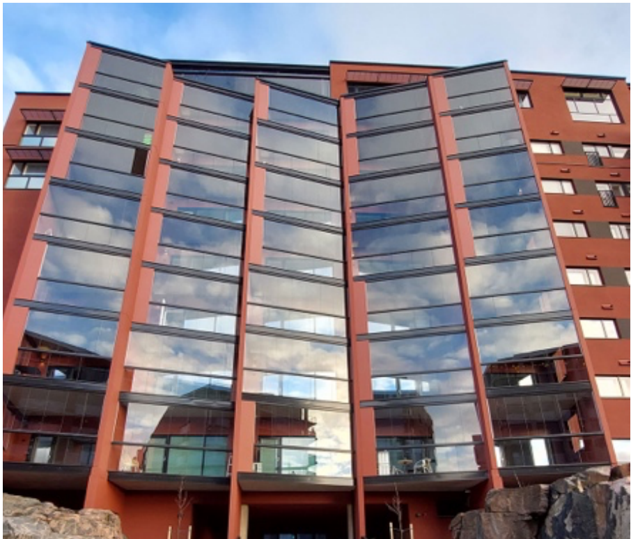
Figure B2 Streetview of the building after adaption. Google Maps (2023).
