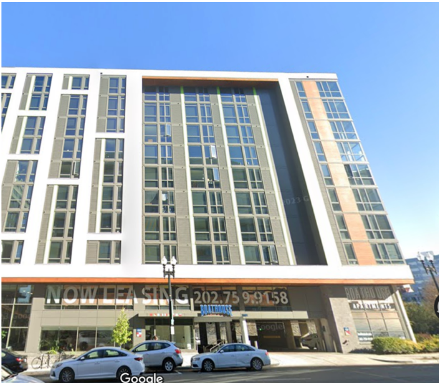
Figure E4 Street view of the building after adaptation. Google Maps (2022).
