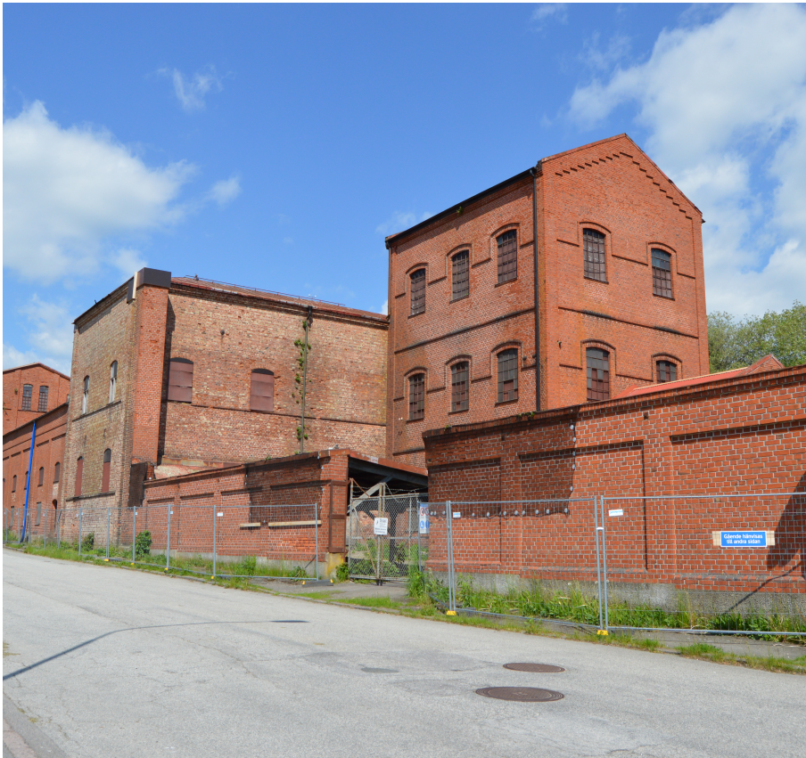
Figure C4 Building before adaptation. Picture by Väsk is licensed under CC BY 4.0.
