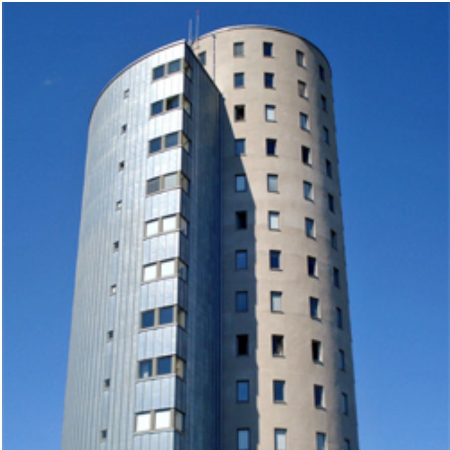
Figure E1 The building after adaptation. Picture by Mangan 2002 licensed under CC BY 3.0.
