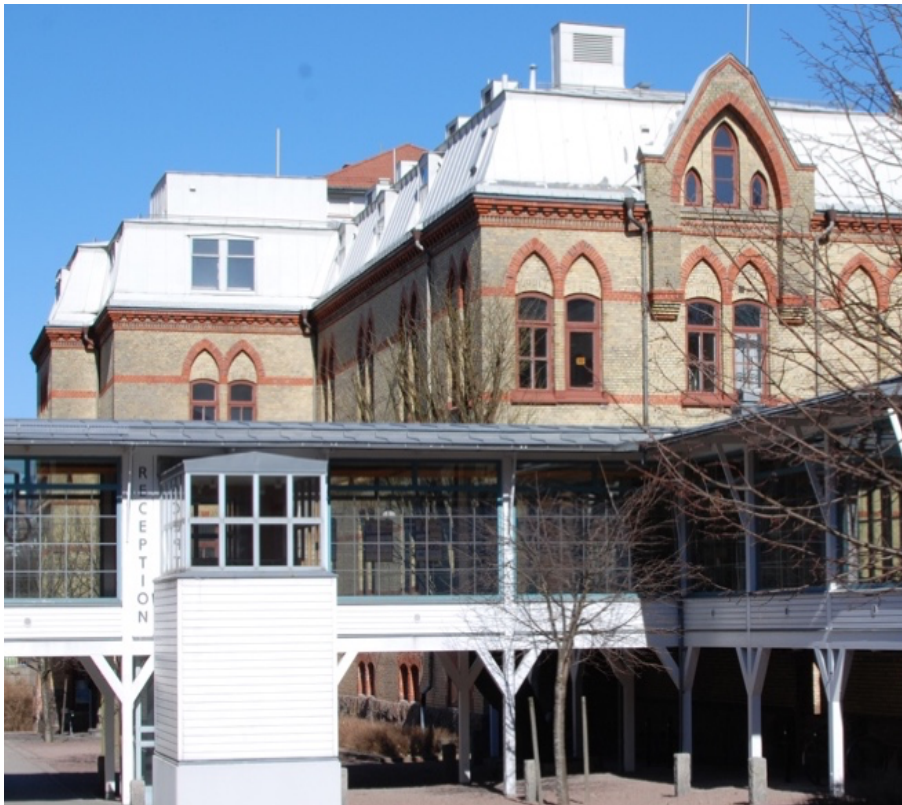
Figure A2 The building before adaption. Photo by Unknown licensed under CC BY.
