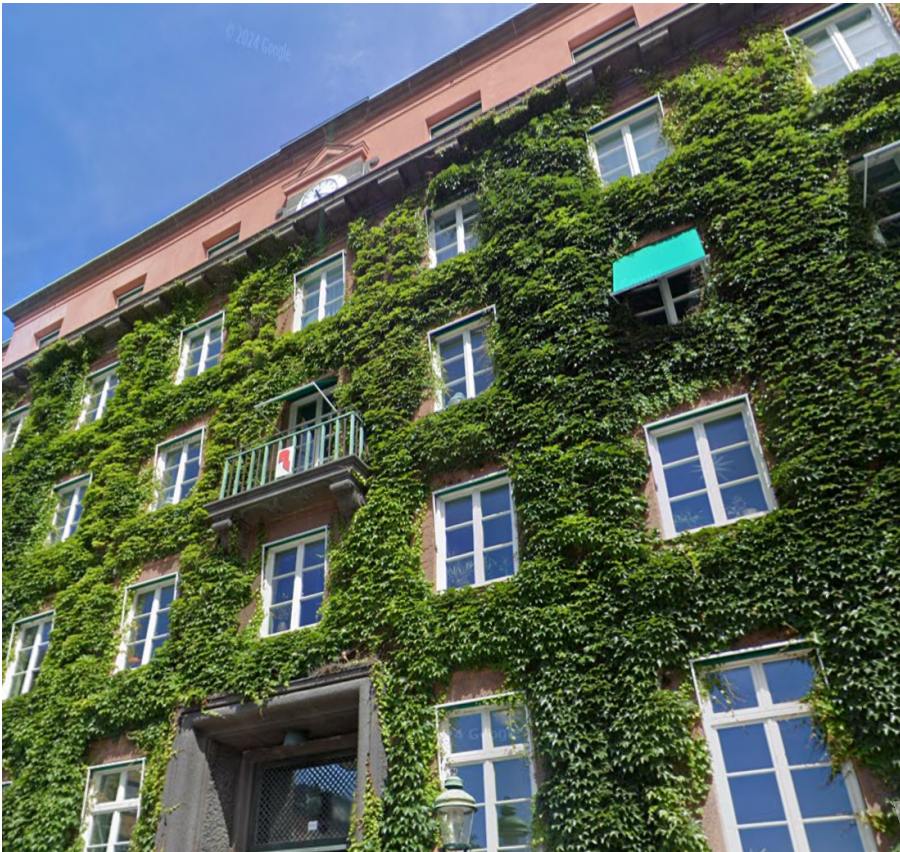
Figure A5 Streetview of the building after adaption. Google Maps (2022).
