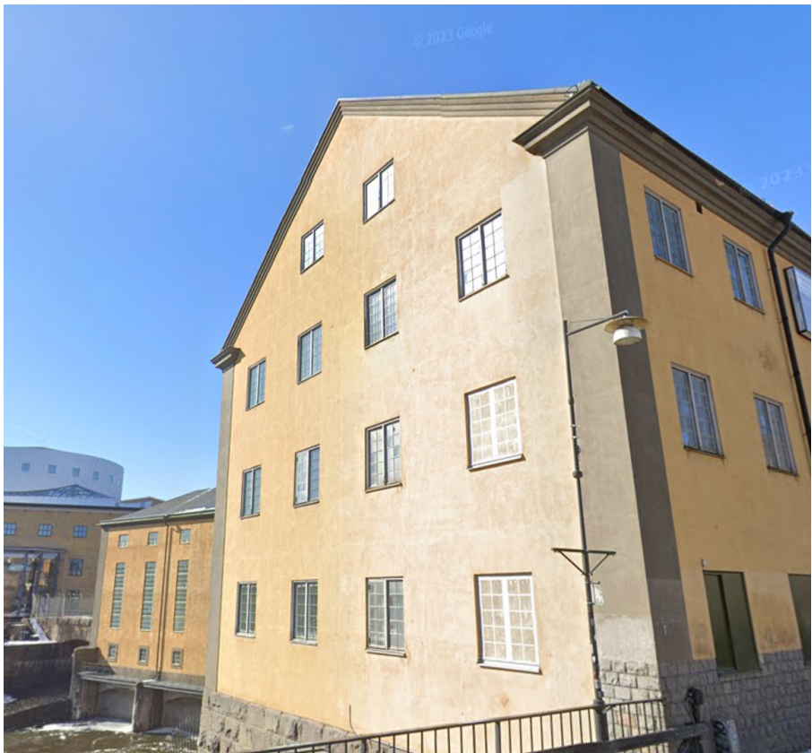
Figure C3 Street view of the industrial site of Yllefabriken. Google Maps (2023)
