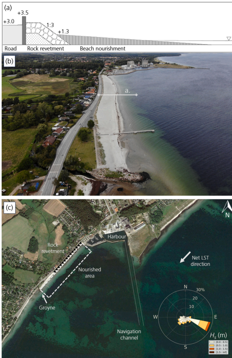
Fig. 2. Overview of the managed coastal stretch. (a) Schematic cross-section of the protection; heights are indicated in m DVR90. (b) Drone image from July 2021, just after completing the nourishment, Photo: Danish Coastal Authority. (c) Satellite image (Google Earth Pro version 7.3.6, image date: 2019/08/25) with important attributes indicated.
