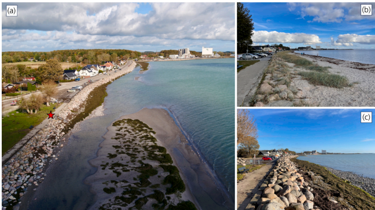
Fig. 10. Images showing the post-storm view of the nourished coastal stretch; (a) drone image from 2023/10/23, Photo: Gregor Luetzenburg (b) before the storm on 2023/10/18, water level is +60 cm, and (c) after the storm on 2023/10/23, water level is +30 cm. The star in (a) indicates the location where pictures (b) and (c) are taken Photo: Anna Adell.
