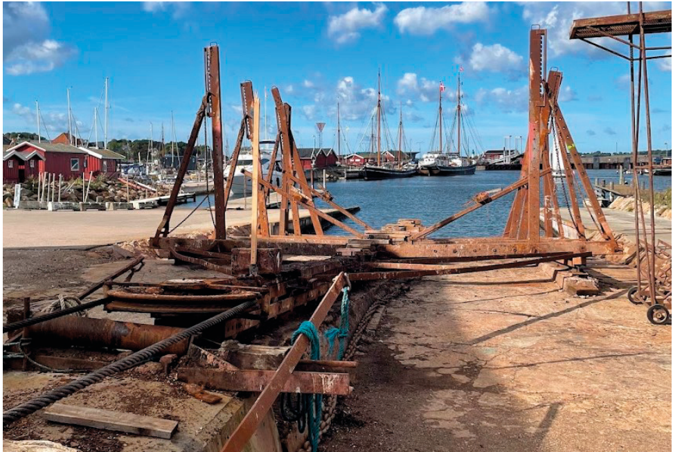
Figure 8 Traditional slipway in Holbæk, Denmark
