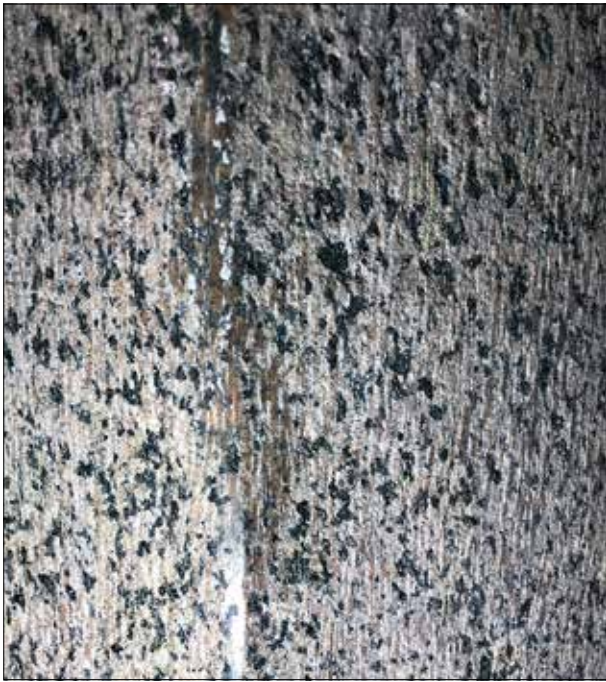
Fig. 6. A close-up of the hexagonal column. The Önnestad syenite has a mixture of black, red and white grains. It has become bleached and greyish over time. Initially the column was highly polished around 1250, as can be seen on the outer edge of all six angles of the hexagonal columns. After a fire around 1320 the surface was damaged and recut with a broad chisel, everywhere except the fragile corners. Photo: Chatarina Ödman 2020.
