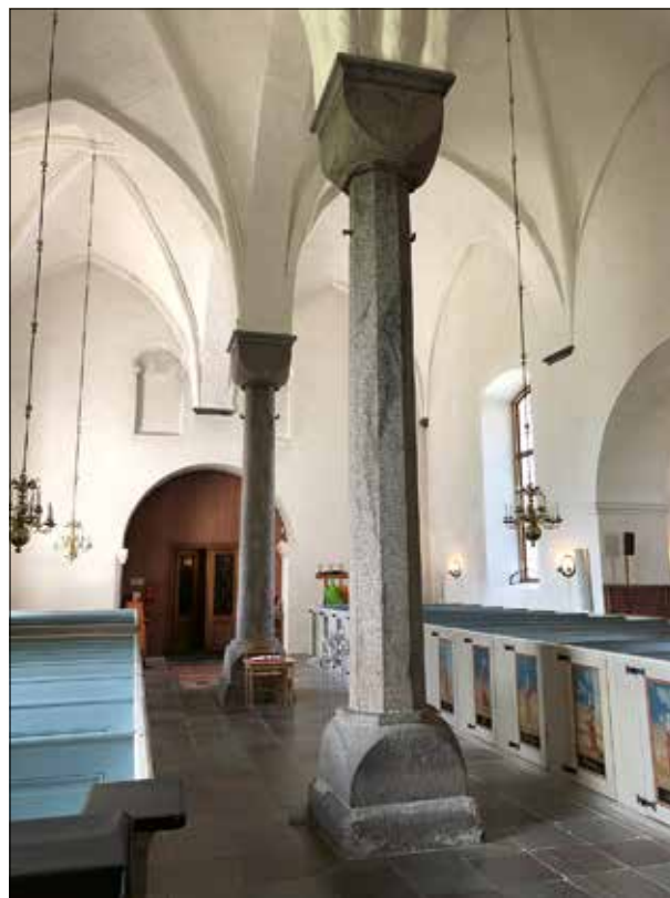
Fig. 4. The nave viewed from the east. In the western wall are the sealed openings to the royal gallery, built around 1121. The two columns, erected around 1250, dominate the space. All parts are made of the same rock. The height is exactly calculated so that the wall arches of the vaults do not cover the openings to the loft. Photo: Chatarina Ödman 2020.
